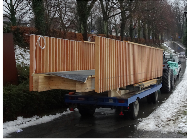
The structure weighting of several tons was delivered ready to drive by a semitrailer truck
