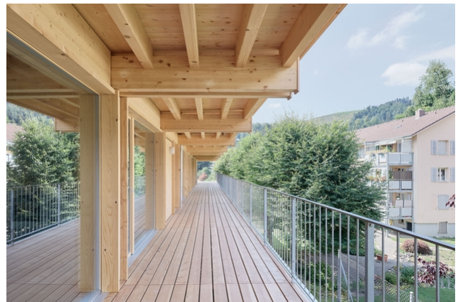
On the pergolas serve to protect the wood and are outdoor space at the same time.
