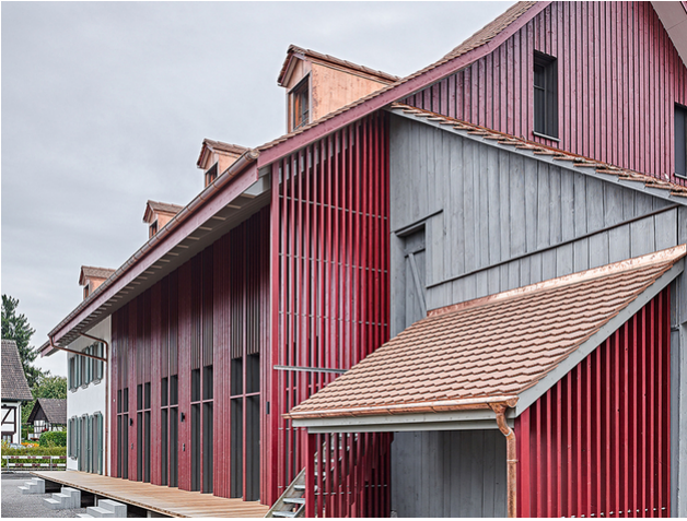
The wooden formwork has been painted with an oxide oil glaze
