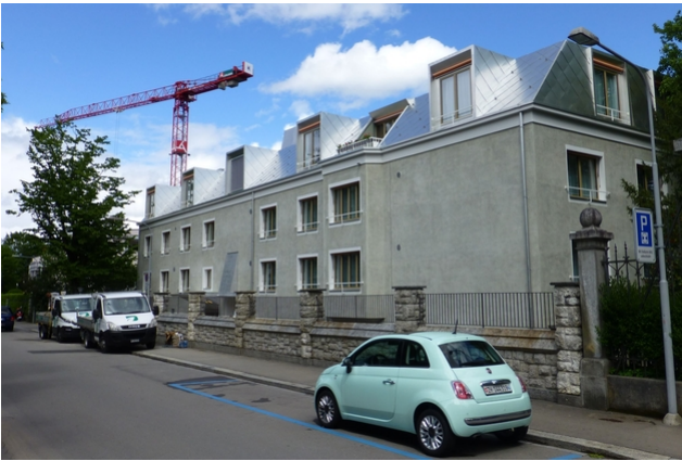
Exterior view in finished state
