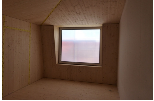
Interior view during the construction phase
