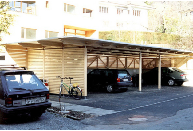
Finished car shelter
