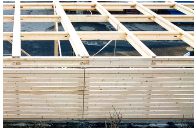
Finished car shelter
