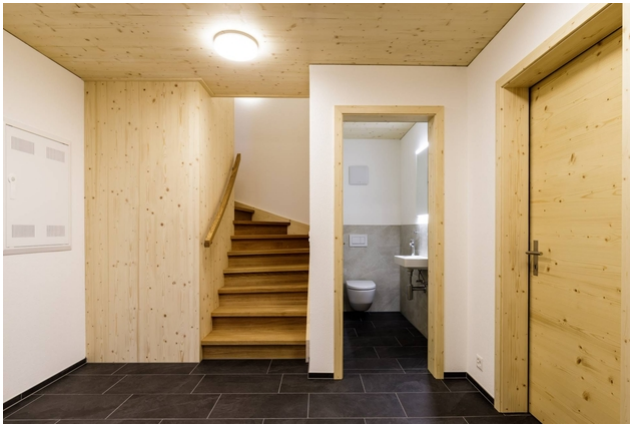
Ceiling insulation in barn conversion.
