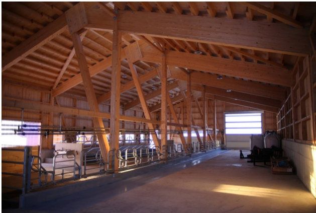
Frame construction in free range barn
