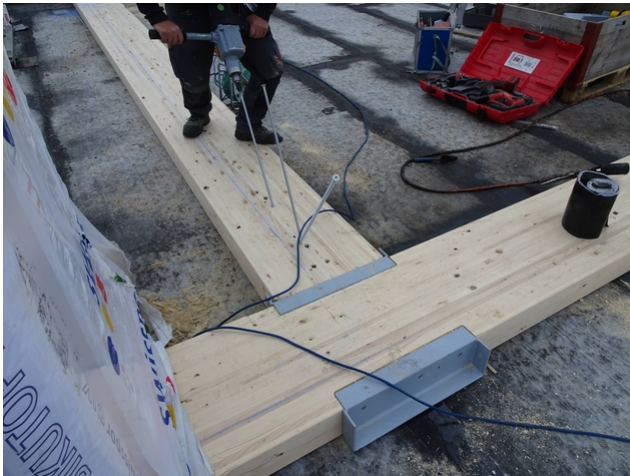
Reinforcement from above
