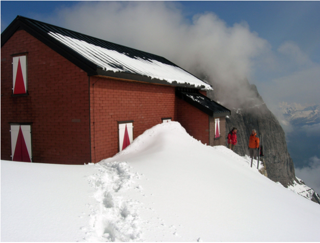
The original Dossen hut
