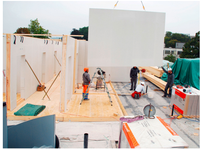
Relocation partition walls addition
