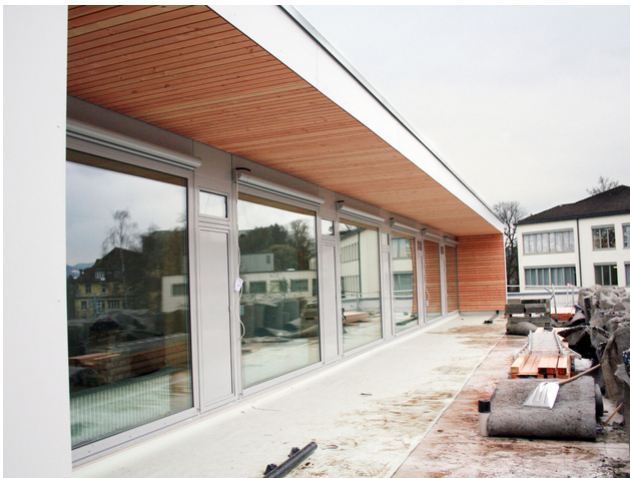
Facade view extension north side
