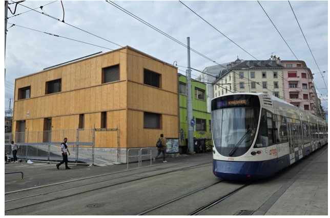
View of the extension from the north
