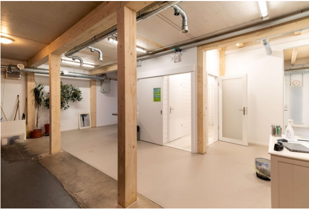
Central post-and-beam structure
