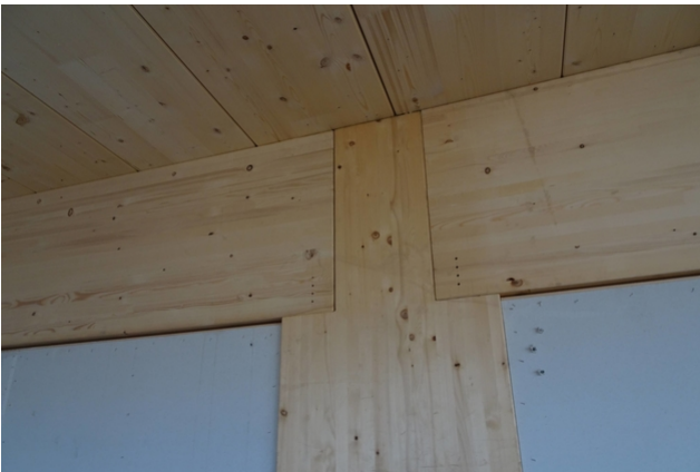
Bearing of the beams on the supports
