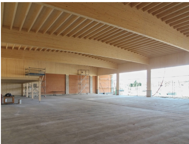
View inside: The 25 meter long trusses support the hall roof
