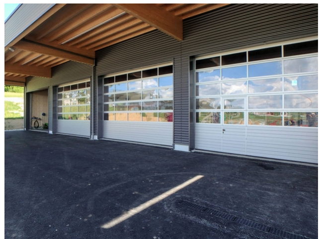
The canopy of the new garage is a proud 5 meters wide
