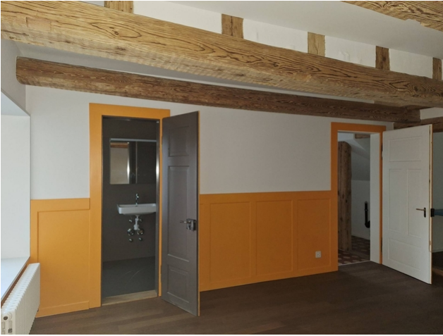
The floor slabs were carefully reinforced, restoring parts of the existing structure to their former glory.
