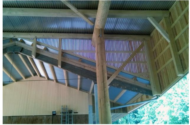
Supporting structure in the finished building
