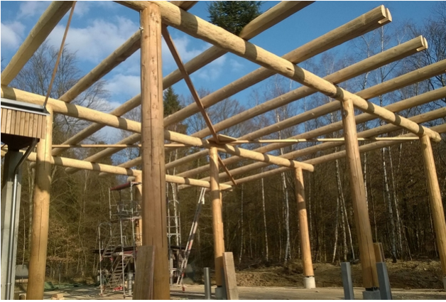
Supporting structure after assembly
