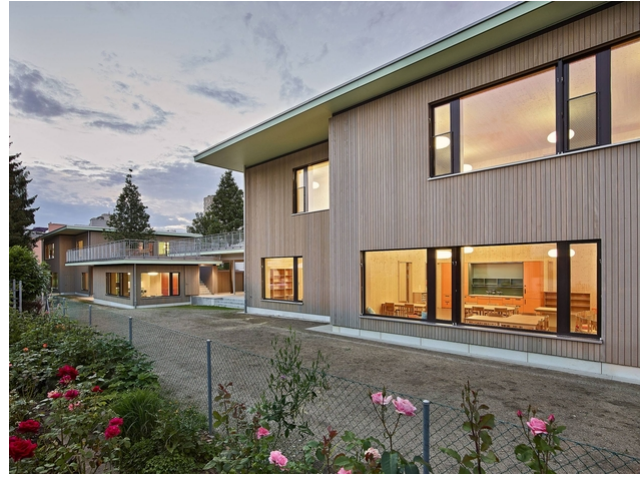
The new kindergarten complex consists of several wooden houses (Photos: Zeljko Gataric)
