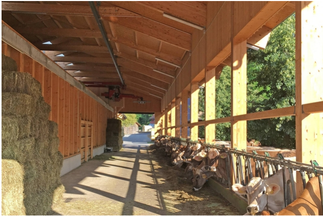
Interior view feed store
