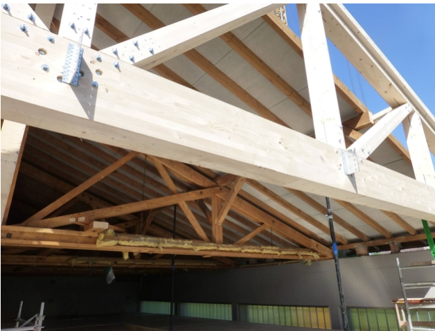
Old and new truss
