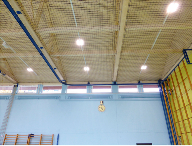
Interior view ceiling
