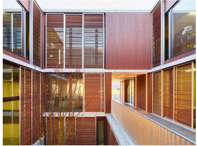
View into the inner courtyard: Filigree wooden sliding elements protect from the sun
