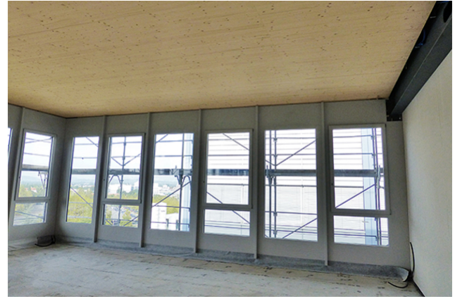
Wooden ceiling with 9m span
