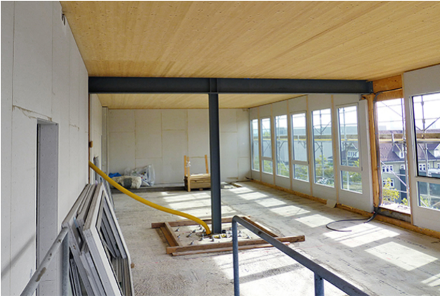
Primary steel structure
