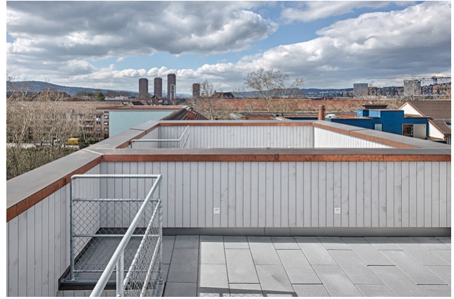
Roof terrace (Photos: Roger Frei Zurich)
