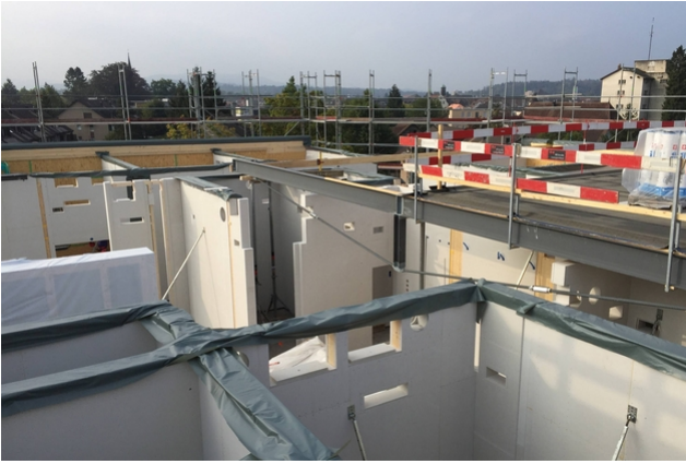
Installation of the under-tensioned beam
