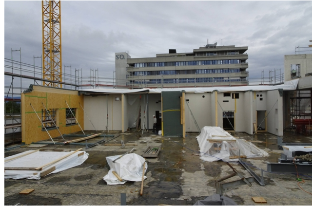
Erected interior wall elements with the prepared recesses for the many installations
