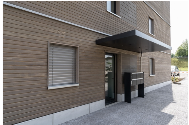
Wooden facade in the entrance area
