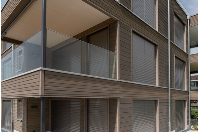
Wooden facade and balconies in the outdoor area
