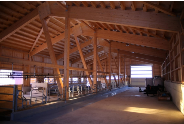
Optimally insulated components ensure a comfortable living environment.
