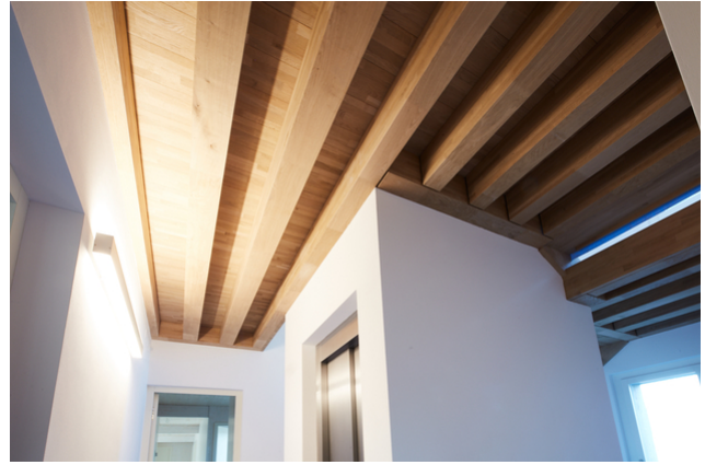
Staircase and elevator shaft in wooden construction
