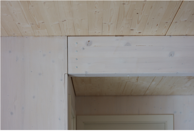
Downstand beam with milled steel plate
