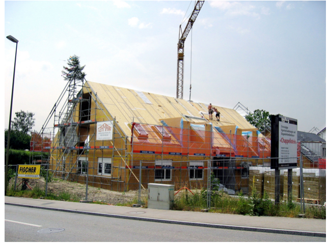
Preparation roof insulation
