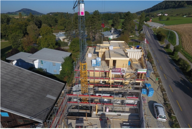
The wooden structure is erected
