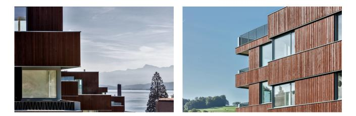
The lightweight timber façade was attached in front of the massive reinforced concrete structure. The wooden façade with sophisticated sheet metal aprons in complex geometries forms the outer shell of this superstructure.
