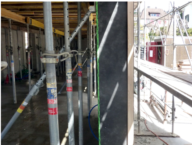
Load-bearing wooden walls ground floor before concreting the ground floor slab
