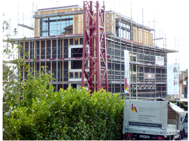
Exterior view from the street side from above in the carcass
