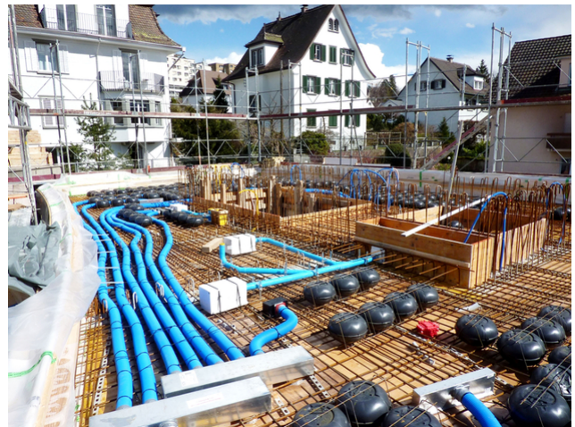
Concrete ceiling over ground floor shortly before concreting
