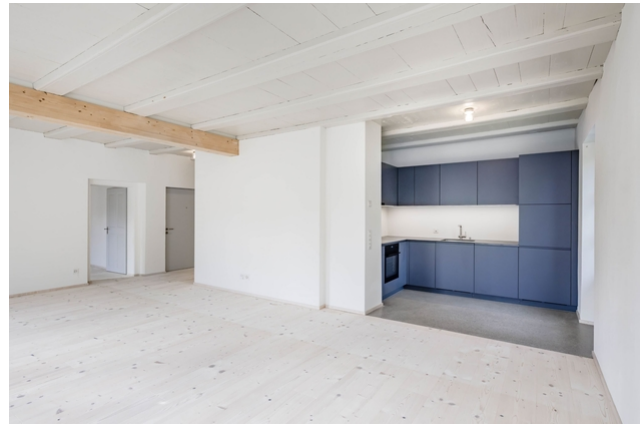
Visible bottom chord of the Vierendeel girder
