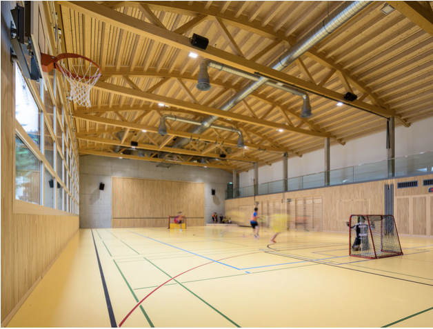
View into the 28 meter long hall. Behind the wooden wall is the stage
