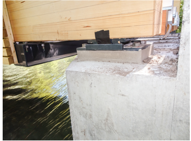
The new bridge was mounted on the existing abutments
