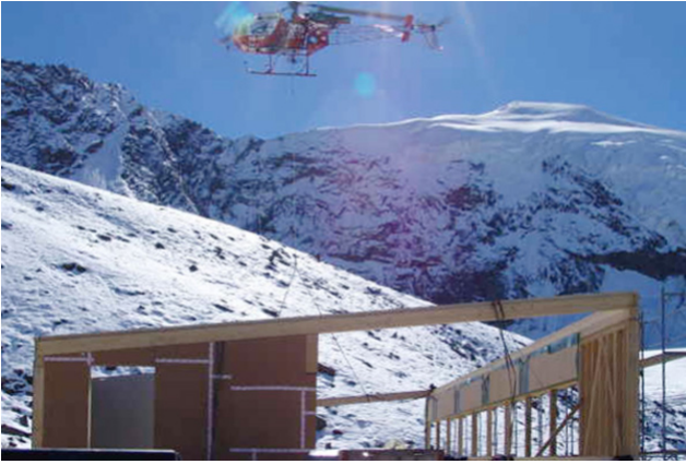
Erection with helicopter
