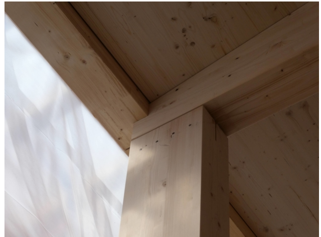
Support beam on support
