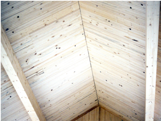
Roof construction with optiholz board stack modules
