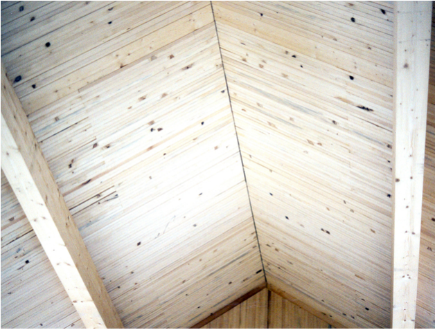
Roof construction with optiholz board stack modules
