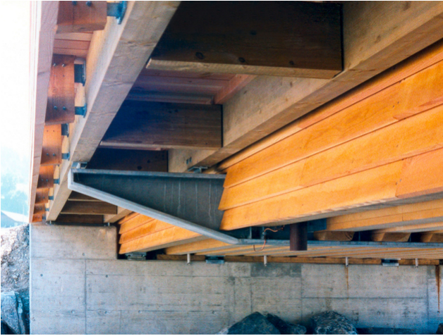
Built-in steel cross member
