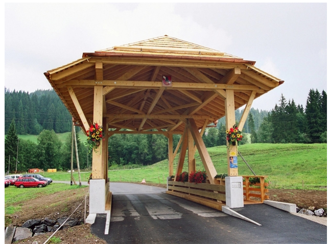
View of the bridge
