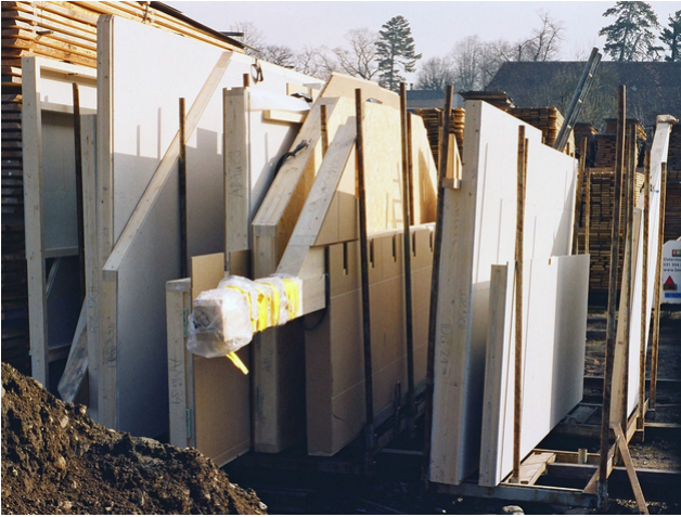
Storage of the walls
