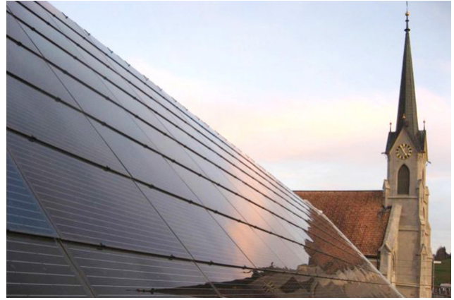
Wooden element roof with photovoltaic system for electricity generation
