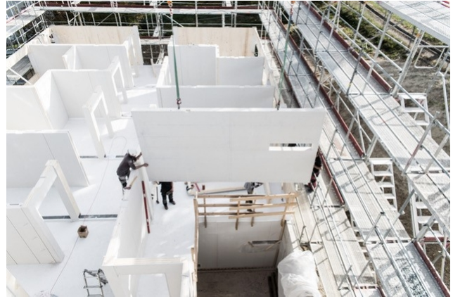
Assembly of the interior walls forming the fire compartment
