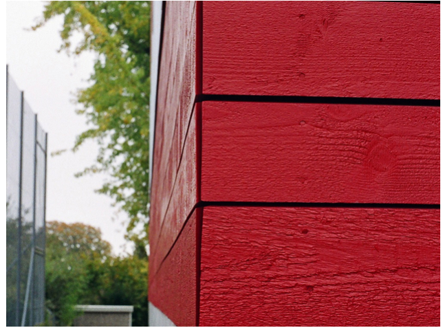
Formwork corner area
