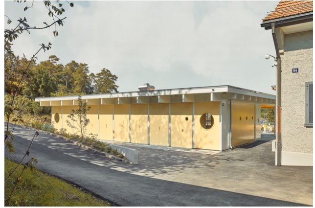
A large canopy for protection from the weather
