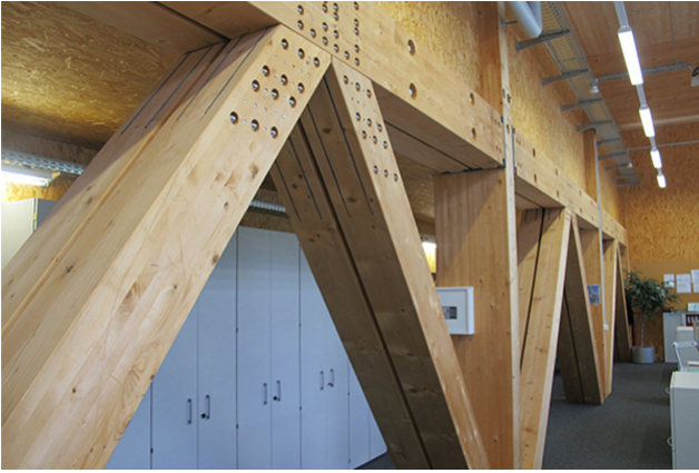
Truss in office wing
