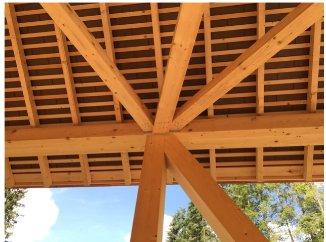
Half timber node: two truss structures converge here
