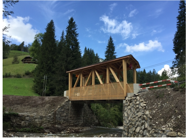
Instead of a concrete bridge, there is a new wooden bridge in the Bernese Forest
