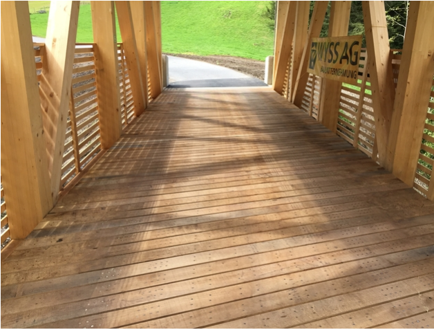
All wood: the flooring of the bridge is made of oak planks
