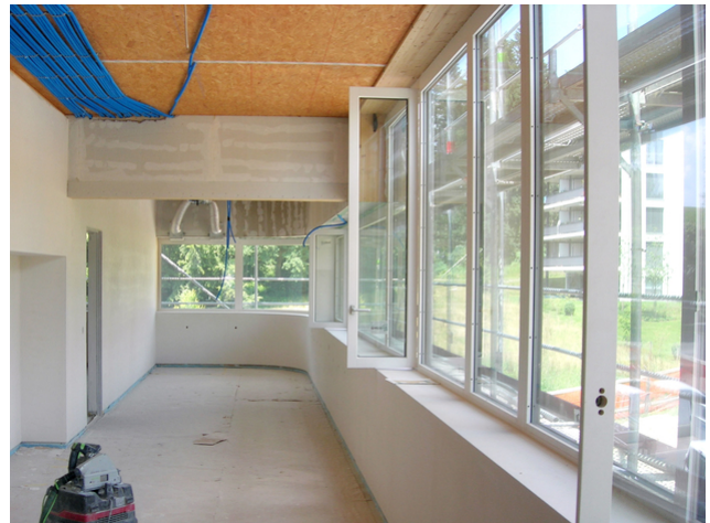
Work niche with cantilevered BSH beam
