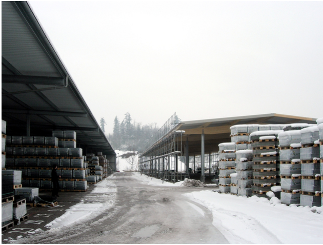
Old and new roofing
