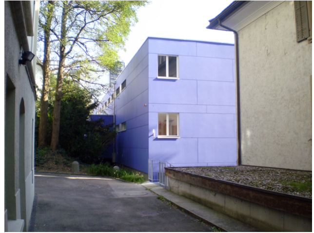
Front view with entrance front
