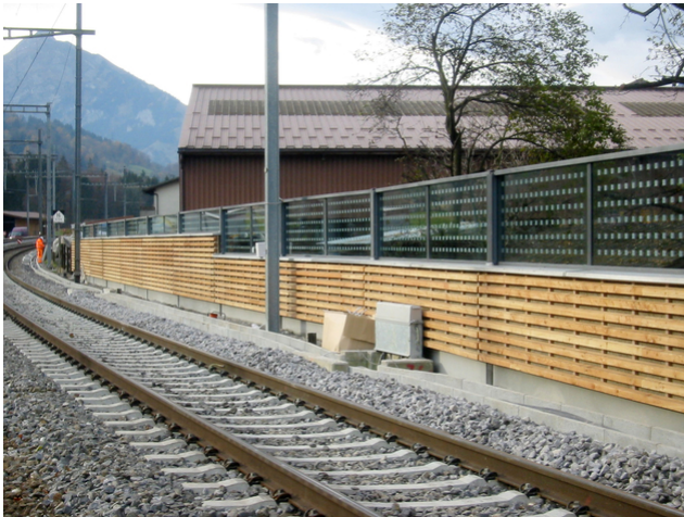
View from the track side
