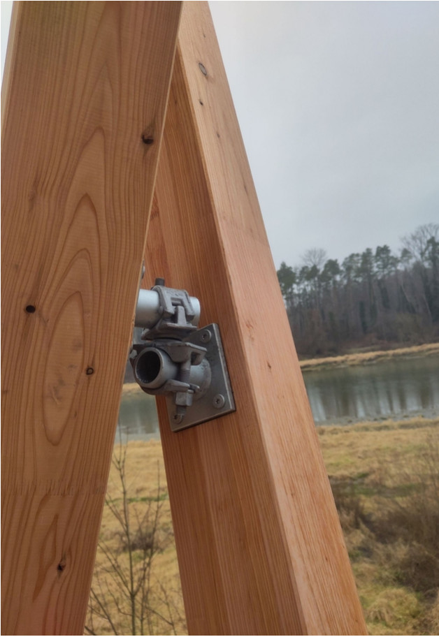
Connection of the lattice bars
